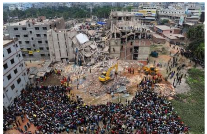
Aerial view of the Rana Plaza Building following its collapse in April 2013. Source: Guardian/Munir Uz Zaman/AFP/Getty Images
